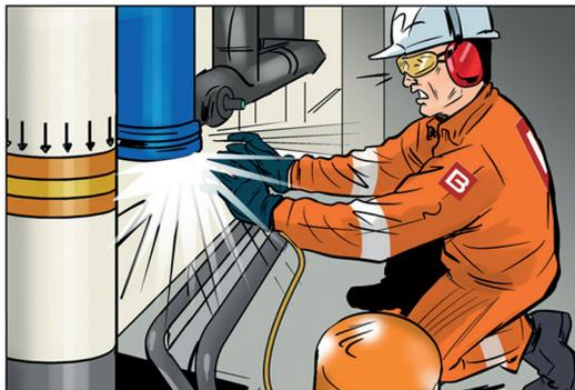
**LA VANNE ÉTANT MAL FERMÉE, LE GAZ JAILLIT ET LE CHEF MÉCANICIEN SE BRÛLE GRAVEMENT EN ESSAYANT DE STOPPER LA FUITE AVEC SES MAINS.**
