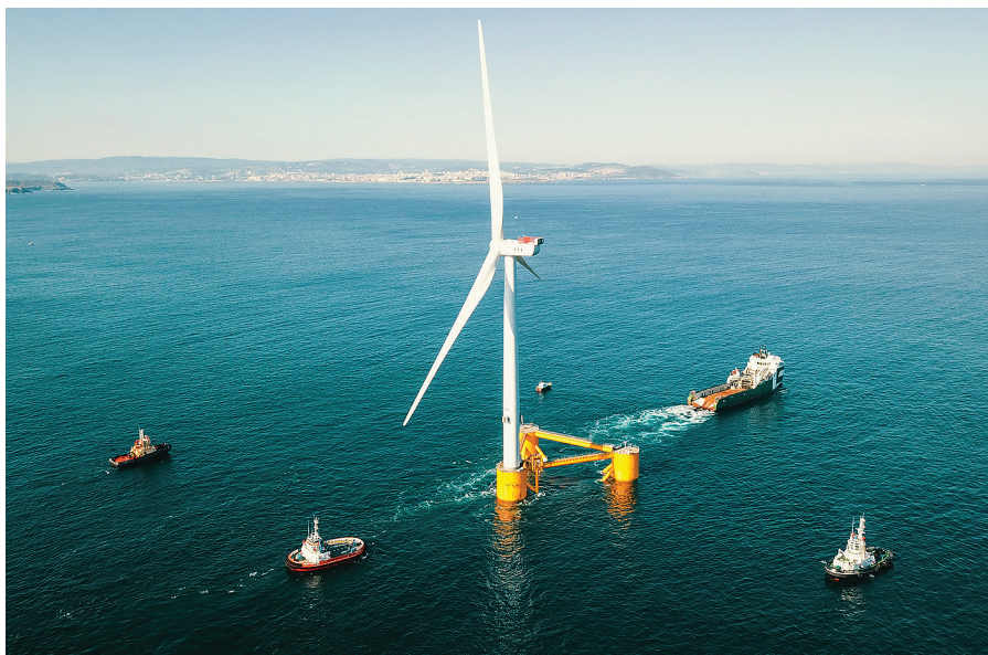
Fig. 3. The Bourbon Orca, flagship of the Bourbon fleet, tows the third floating wind turbine of the WindFloat Atlantic project, off the Portuguese coast.
