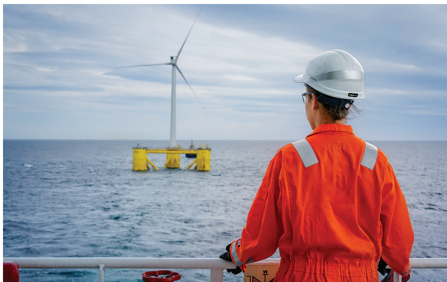
Fig. 1. The towers of the wind turbines are 100 m tall, the rotor assemblies are 164 m in diameter, and the floaters are 30 m tall. The wind farm is located roughly 20 km out to sea.
